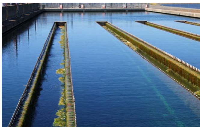
California – Water treatment plant ©Flickr/Aquafornia – Chris Asahin
